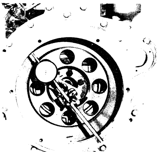
Checking Alignment of Flywheel Housing Bore. P4
